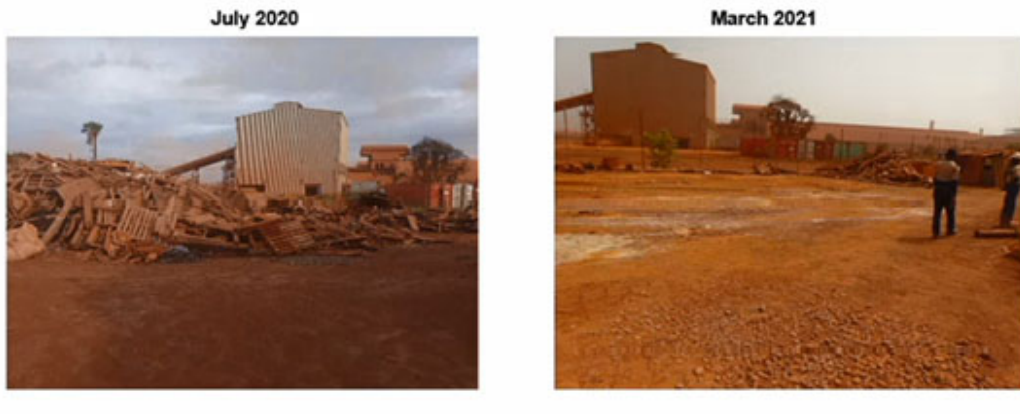
Figure 7-2: Progress with the removal of waste from temporary storage areas
