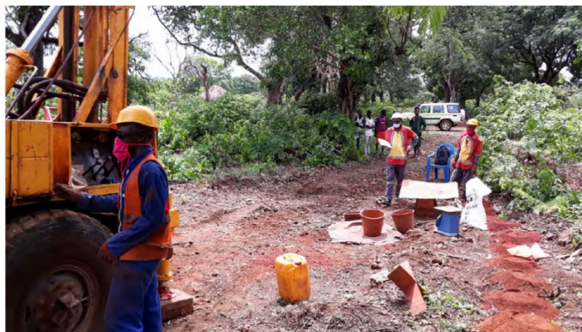
Figure 3-5: Typical layout of drilling location (showing access track and part of drilling rig to the left)
