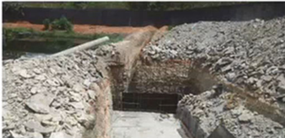
Figure 7-1: Foundations for the UV Wastewater treatment in Sangarédi
