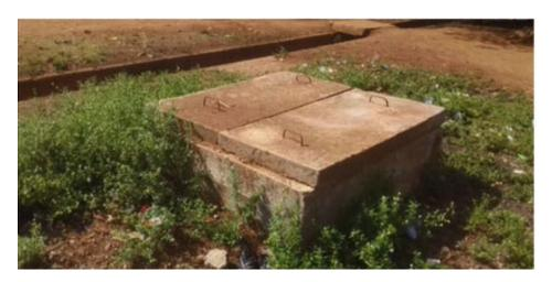
Figure 7-9. Raised and repaired manhole cover to prevent rainwater ingress
