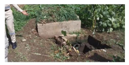
Figure 7-8. Damaged manhole prone to rainwater ingress
