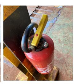
Figure 6-4 Damaged controller module of a lifting device / fire hose cabinet out of order / extinguisher without safety pin
