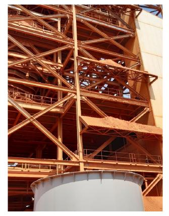
Figure 6-3. Accumulations of dust above a working area
