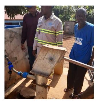
Photo 14. Water pump at Fassaly Foutabhé village with iron removal device to the left
