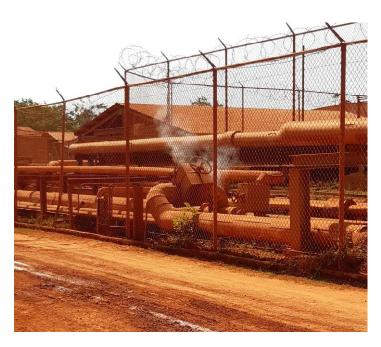
**Photo 12.** Steam from a leaking valve/damaged flange presenting risk to workers
