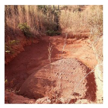
**Photo 17.** Remedial works – enlargement of sedimentation ponds (to prevent sedimentation of nearby watercourse)
