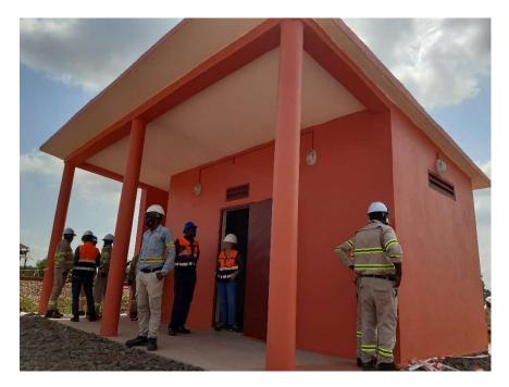
**Photo 21.** Newly constructed bungalow (for signalling equipment as part of MUOA project)
