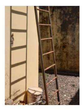
**Photo 13.** Inappropriate fixed ladder for access to roof at the air quality monitoring station, Kamsar
