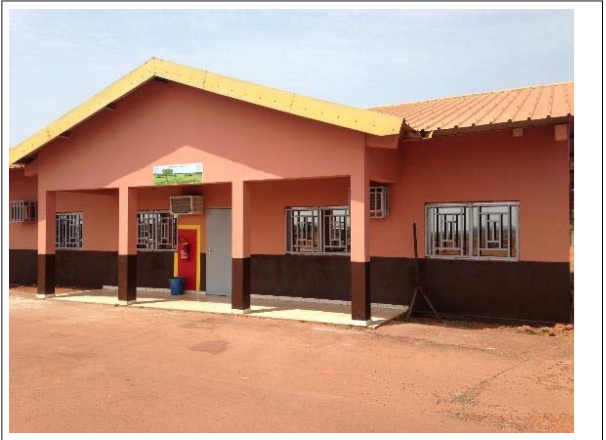
Figure 19: CBG Biodiversity Office at N'Dangara Facility, Sangaredi
