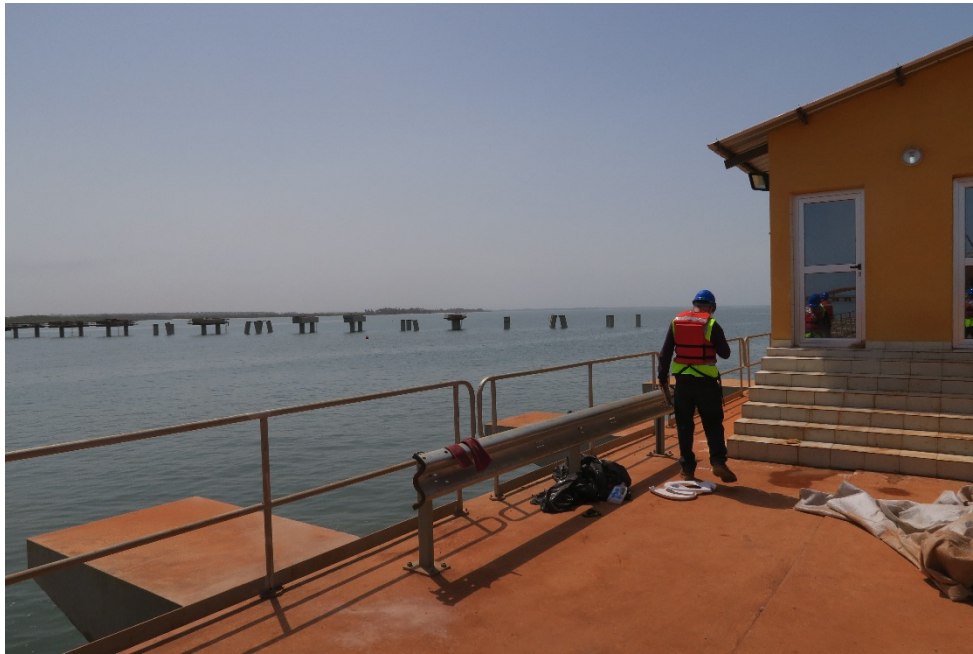
Photo 15. CBG office at end of the jetty - piles for GAC jetty in the background
