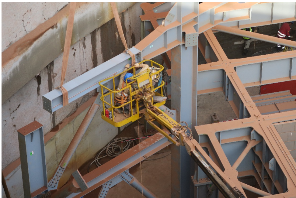
Photo 4. Working at height – good use of harnesses
