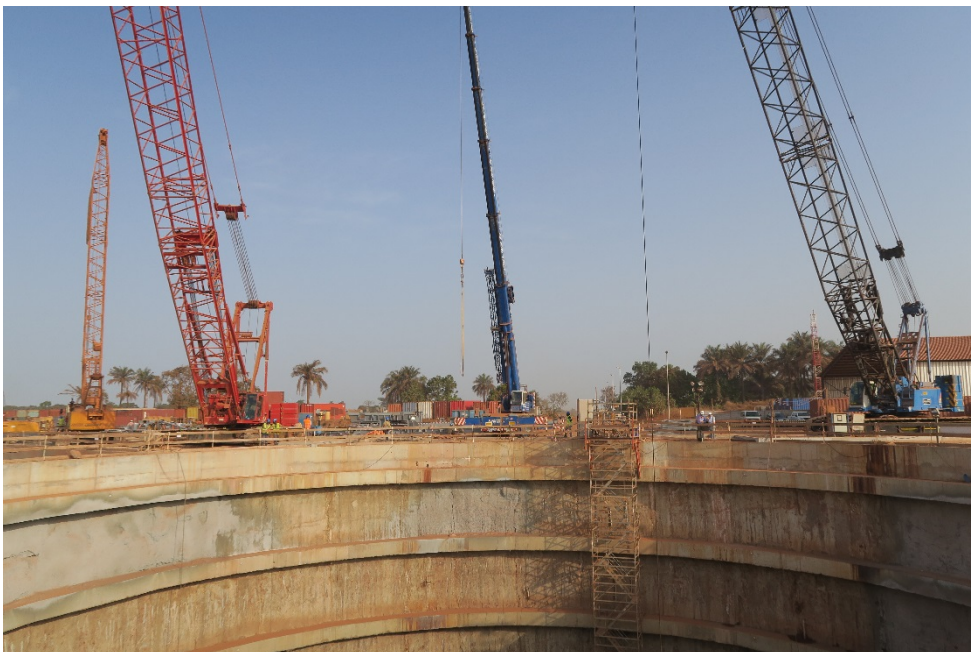
Photo 2. Primary crusher pit – manned access scaffolding on the far side
