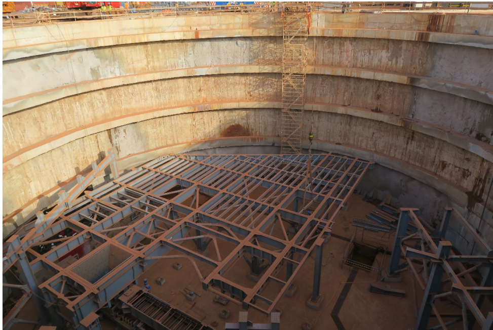
Photo 3. Primary crusher pit – installation of steel work
