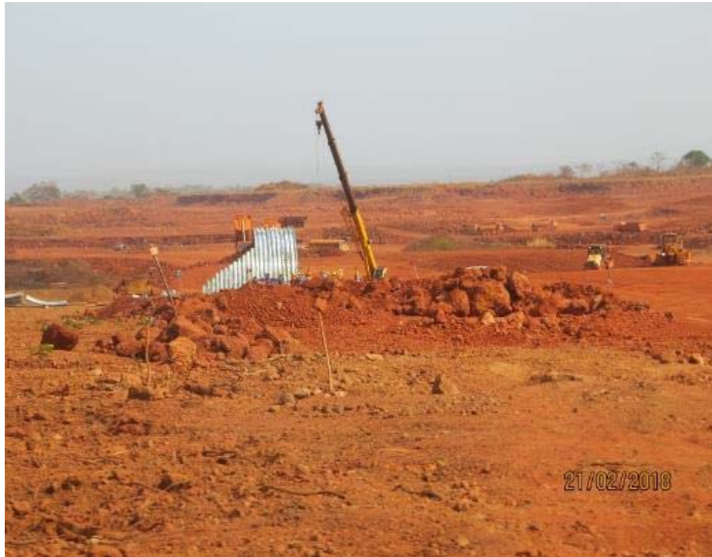
Figure 14: Section of road/rail crossing works near Hamdallaye (close-up)
