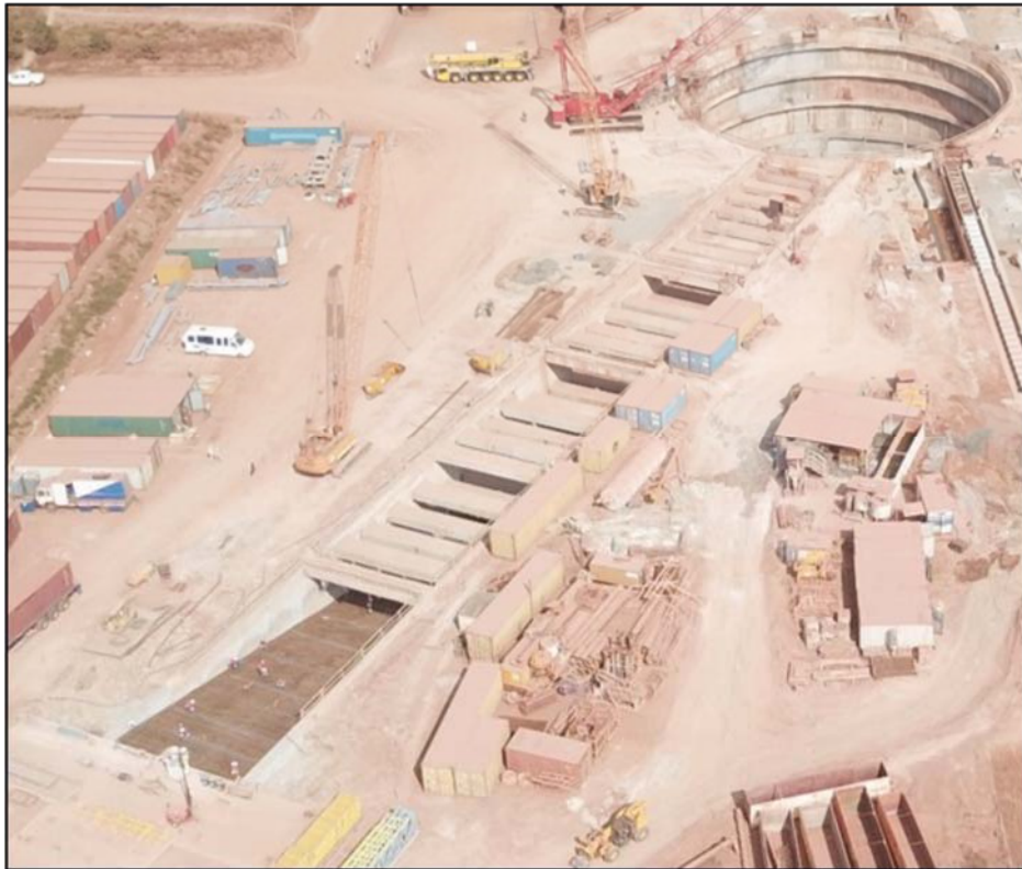
Figure 2: Crusher pit and conveyor trench (courtesy of CBG)
