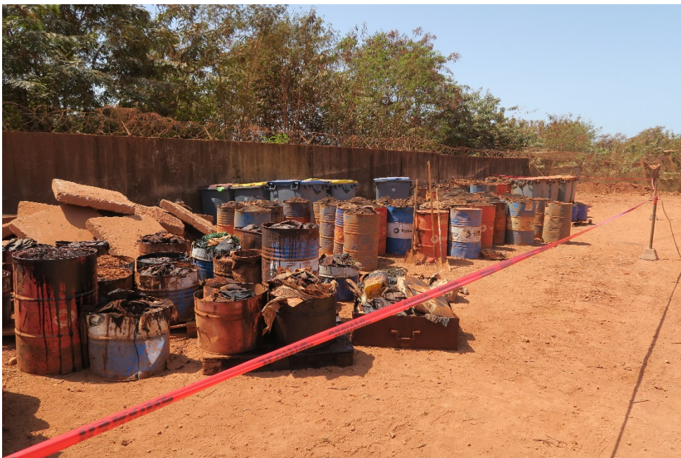
Photo 26. Temporary storage of recovered oily waste following clean up of the creek
