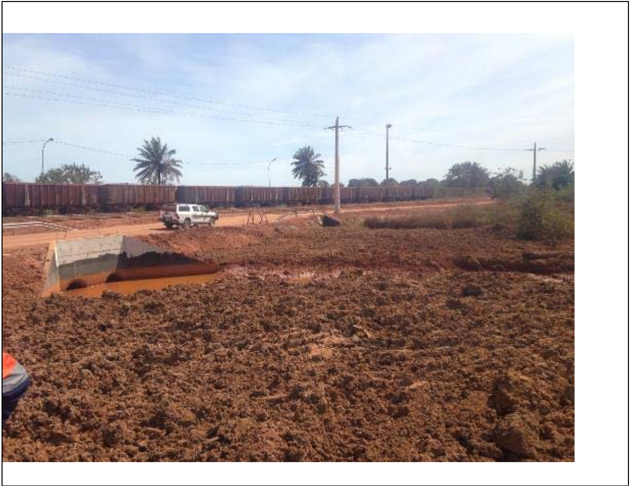
Figure 25: Area of Damaged Mangrove
