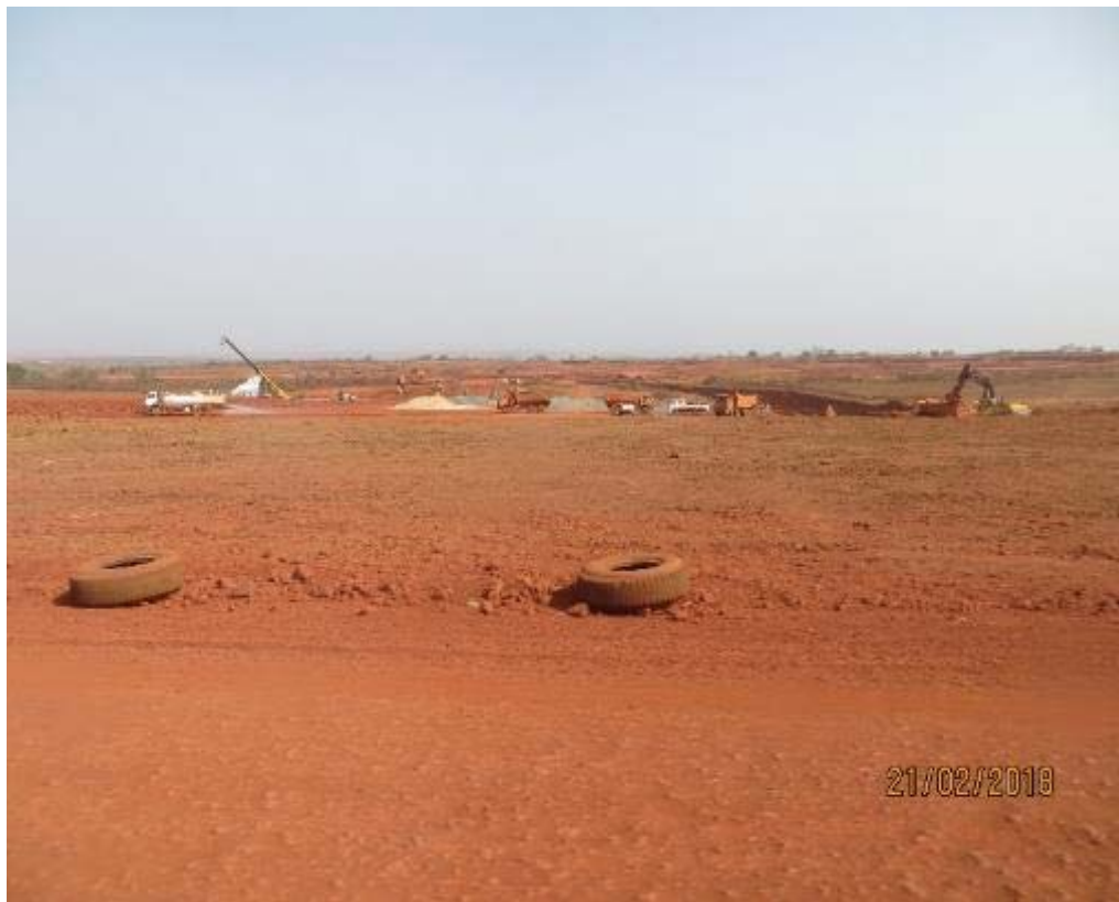
Figure 15: Road/rail crossing works near Hamdallaye (panoramic view)
