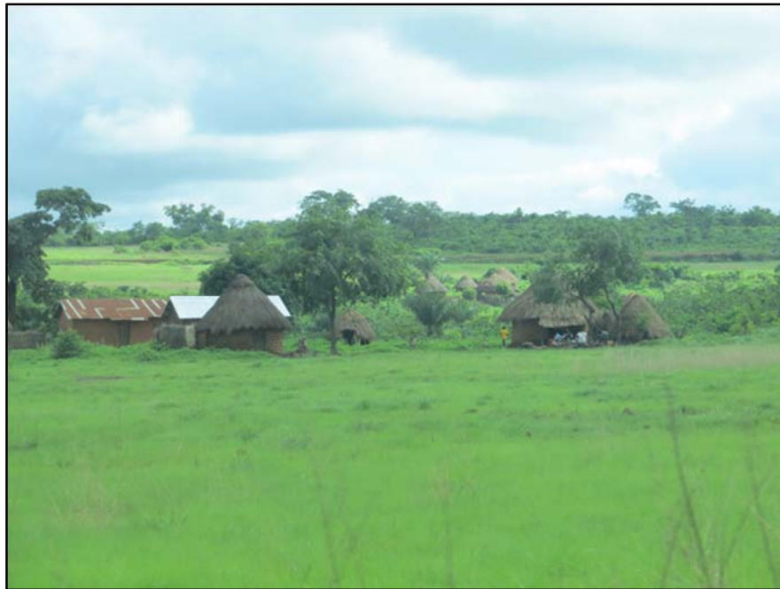
Figure 9-4: 'Hameau' on north side of RN 3 near Hamdallaye. The mix of traditional and modern building materials indicates a degree of investment in the location
