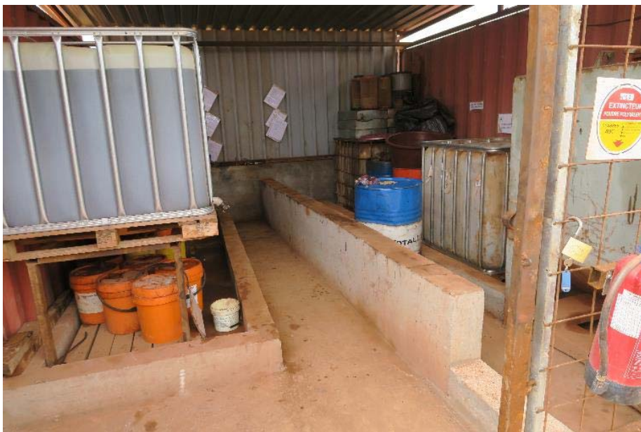
Photo 28. Bunded hazardous liquids and stockpile of hazardous wastes. MSDSs in multiple languages on the wall.
