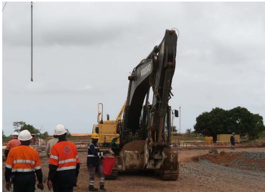
Photo 30. Good practice - moving excavator with flag man
