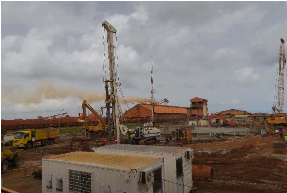
Photo 27. Construction of the new crusher pit at Kamsar
