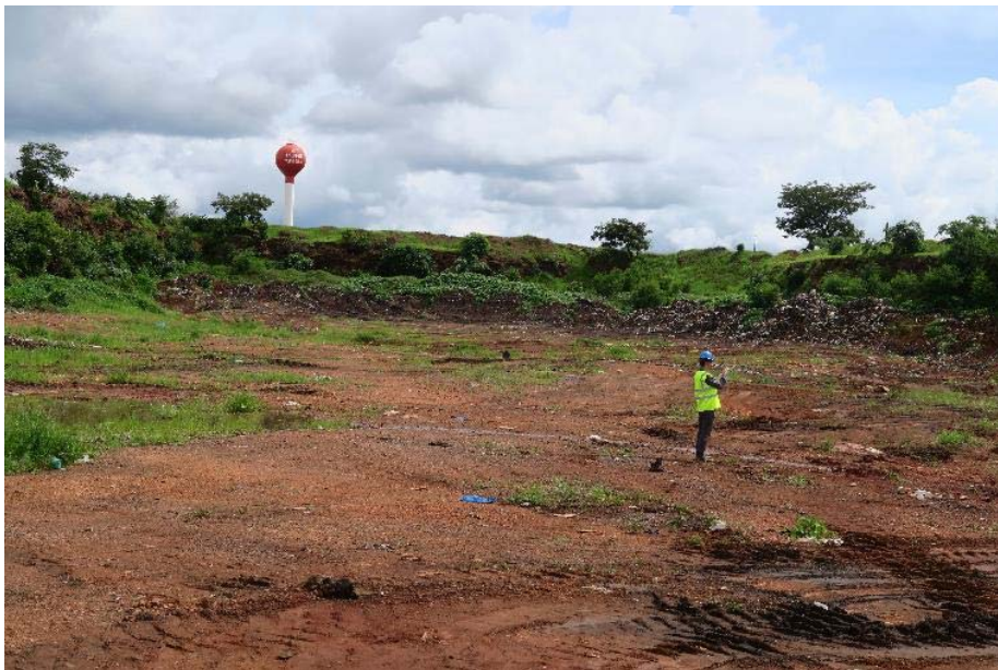
Photo 8. Sangaredi landfill – evidence of some management (compaction and covering with laterite)
