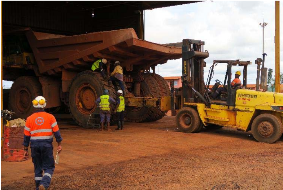
Photo 3. Poor working practices – note use of forklift truck as working platform
