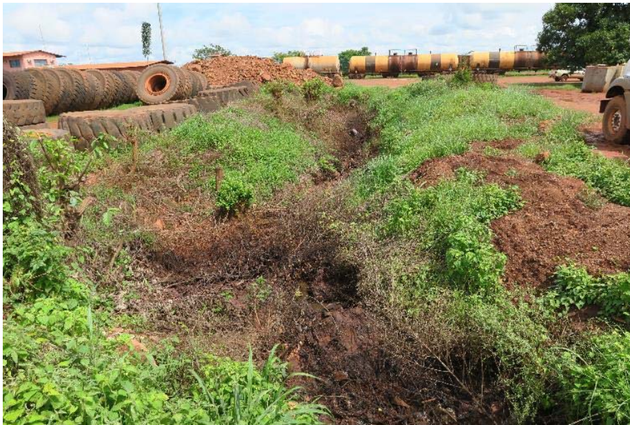
Photo 1. Sangaredi maintenance workshops – oil contaminated drainage channel downstream of oil water separator
