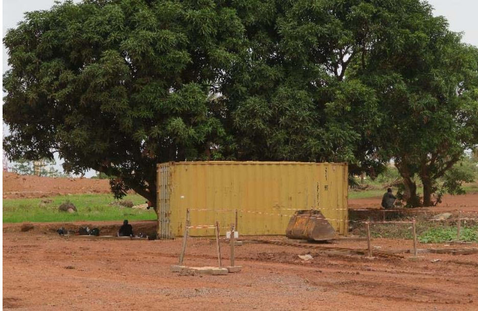
Photo 31. Unauthorised personnel – security and H&S risk
