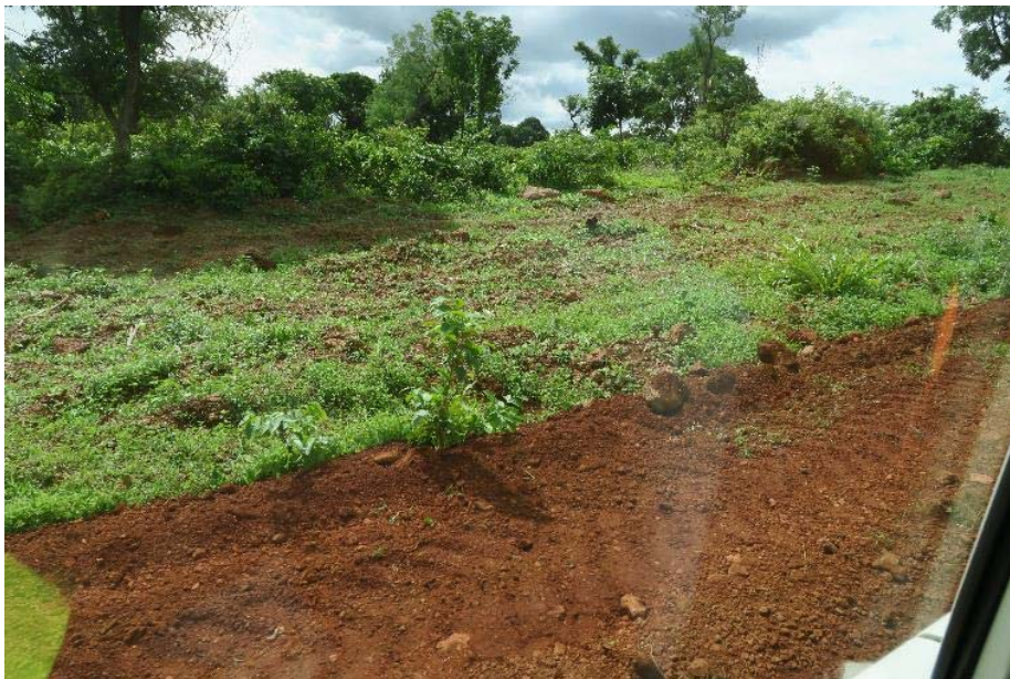
Photo 22. COBAD Road – reinstatement of the abandoned route showing good vegetative cover with onset of rains.
