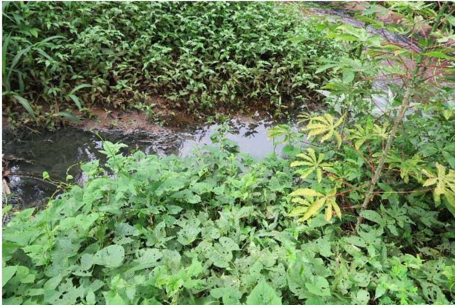
Photo 11. Discharge downstream of Sangaredi WWT plant at confluence with another stream
