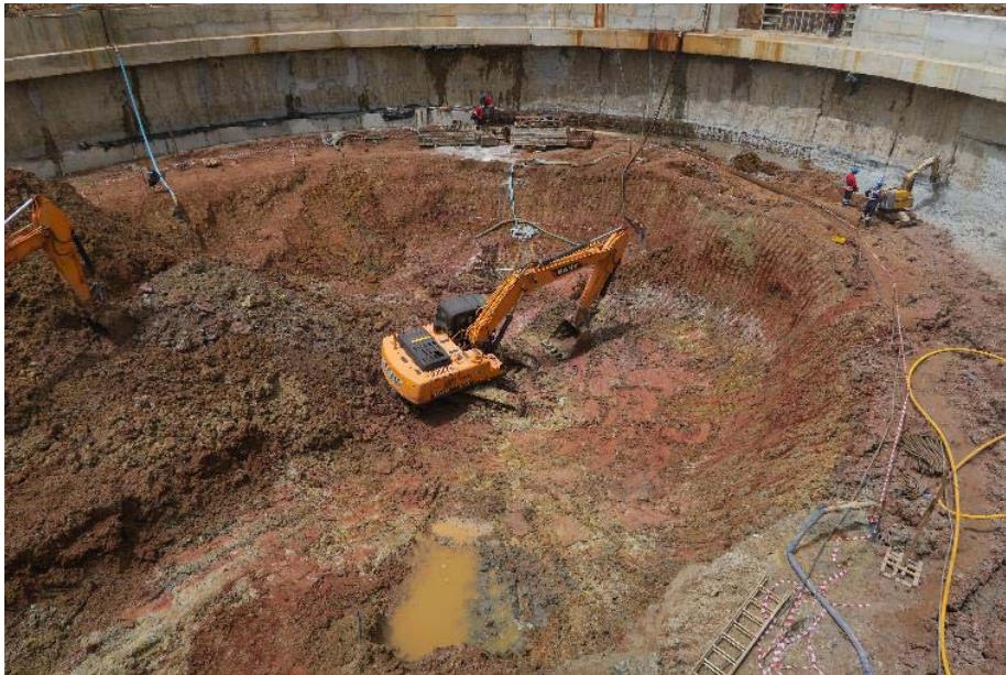
Photo 29. Excavation works inside crusher diaphragm
