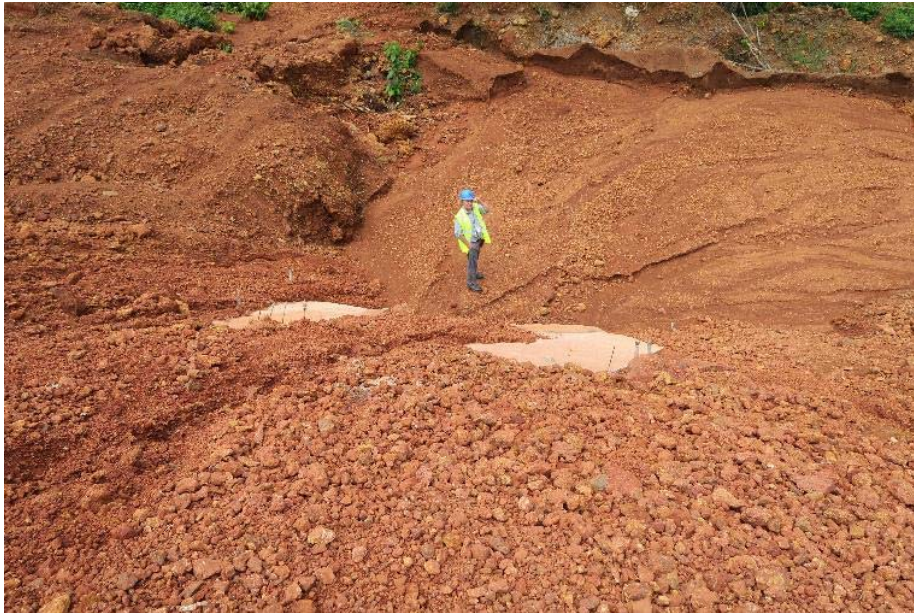
Photo 17. COBAD Road – erosion leading to siltation of watercourses
