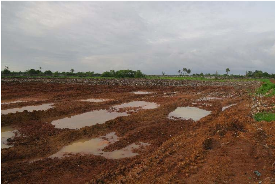
Photo 25. Kamsar Landfill – compaction and spreading of laterite cover with bulldozer
