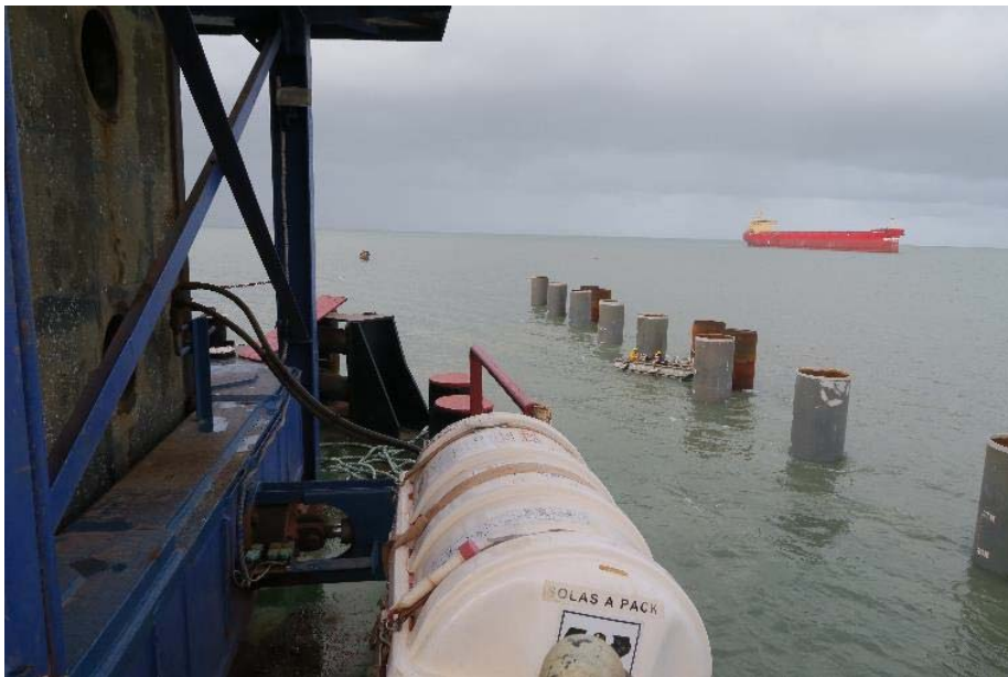
Photo 36. Piles for the jetty
