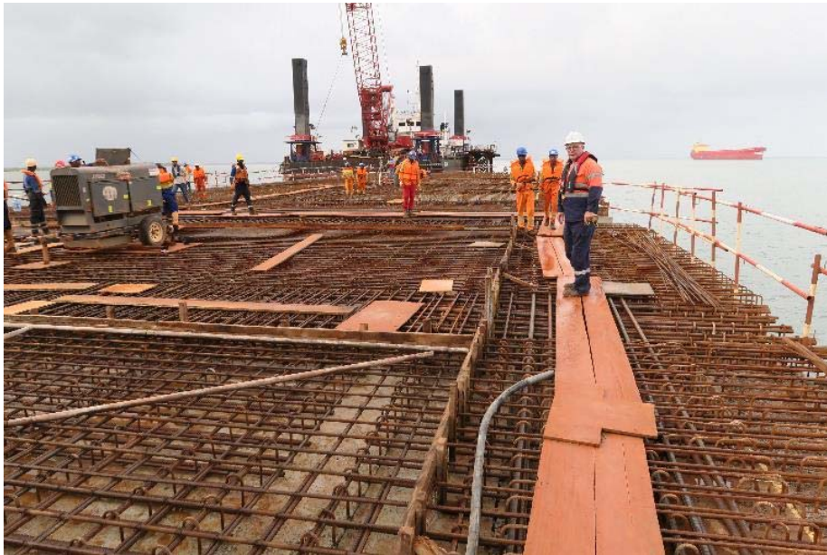
Photo 35. Construction of extended jetty with jack-up piling barge in the background
