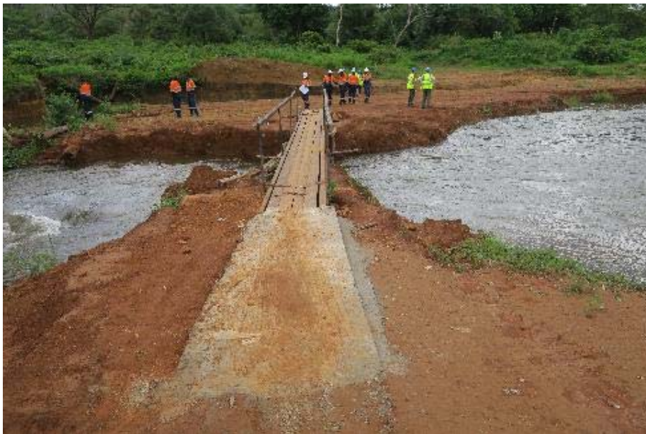
Photo 20. Upgraded temporary foot crossing (replacing earlier log crossing)
