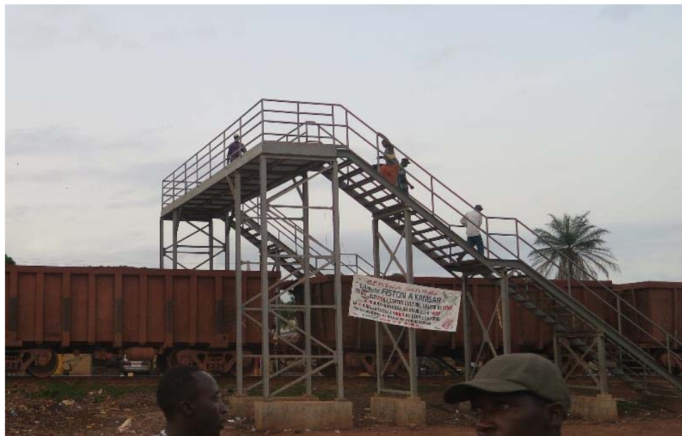
Photo 24. New railway footbridge - in use during passage of trains
