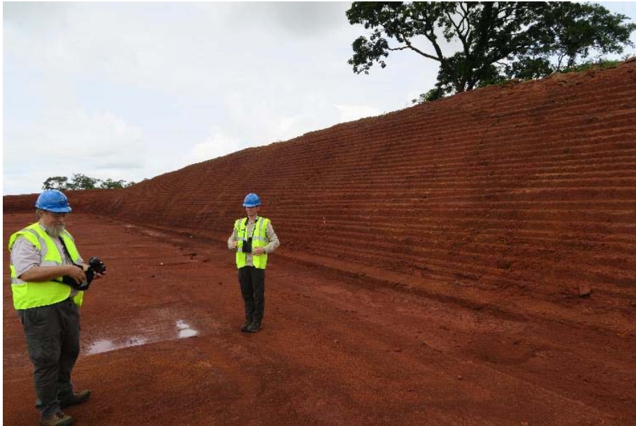
Photo 13. Section 3 of COBAD Road – transfer station. Unprotected steep slopes created by surface miner
