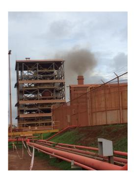
**Photo 10.** New dryer 4 hopper facility (prior to installation of wall panels)
