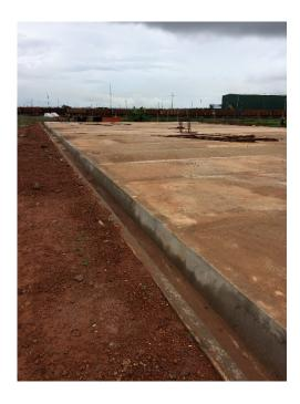
**Photo 4.** Waste reception pad at the Tora Bora waste facility
