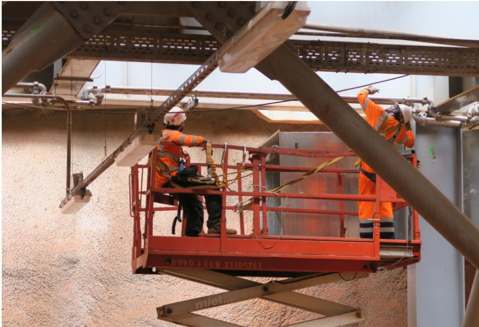
**Photo 5.** Good use of harness and secure lanyard whilst working at height
