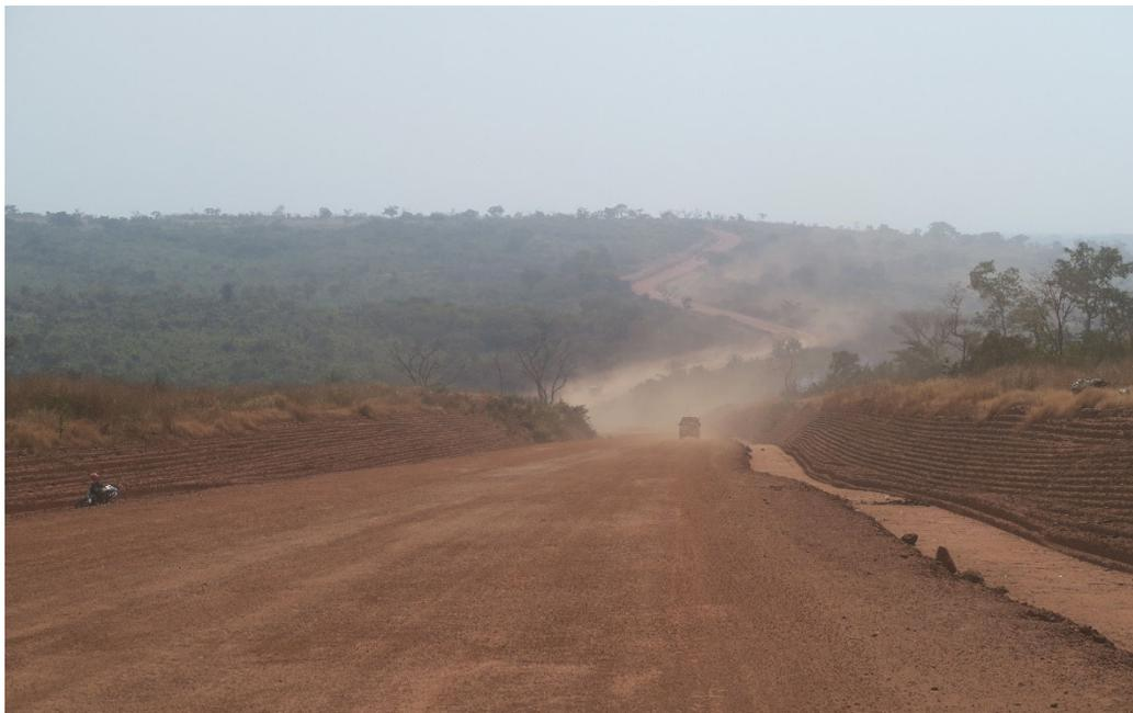
**Photo 35.** Limited evidence of dust control on COBAD Road
