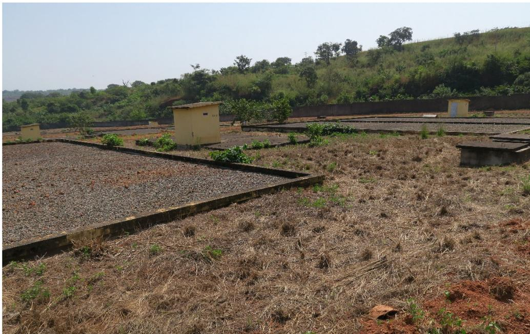
**Photo 28.** Sewage treatment works, Sangaredi. Vegetation removed from filter beds.
