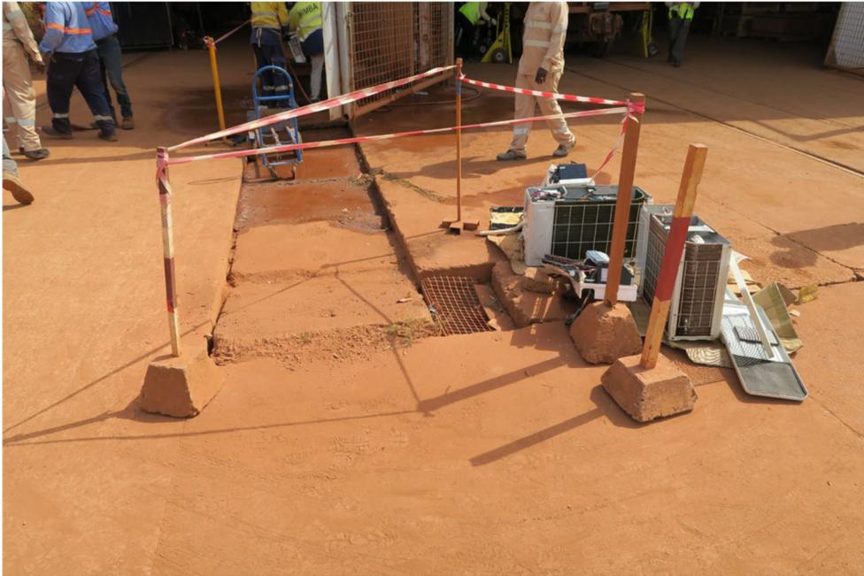
**Photo 25.** Use of simple barrier tape around trip hazard
