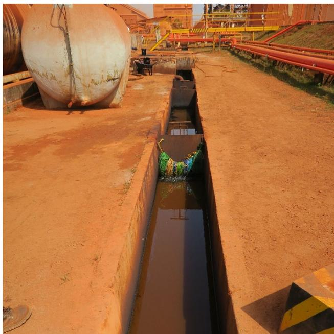
**Photo 20.** Discharge downstream of primary oil water separator
