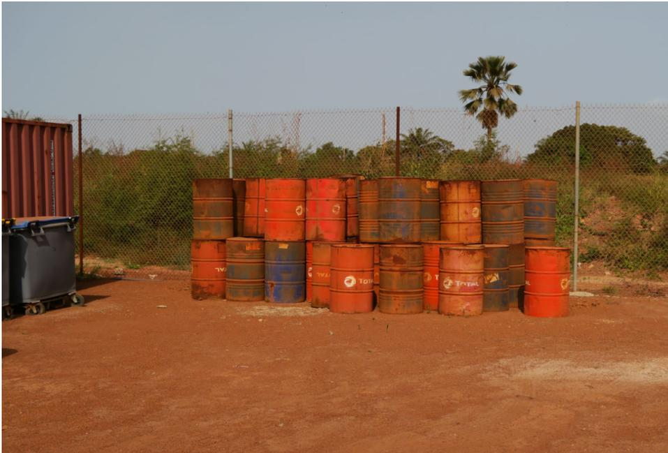
**Photo 11.** Temporary waste storage area (north of secondary crusher) – partial filled drums without secondary containment remain since February 2018
