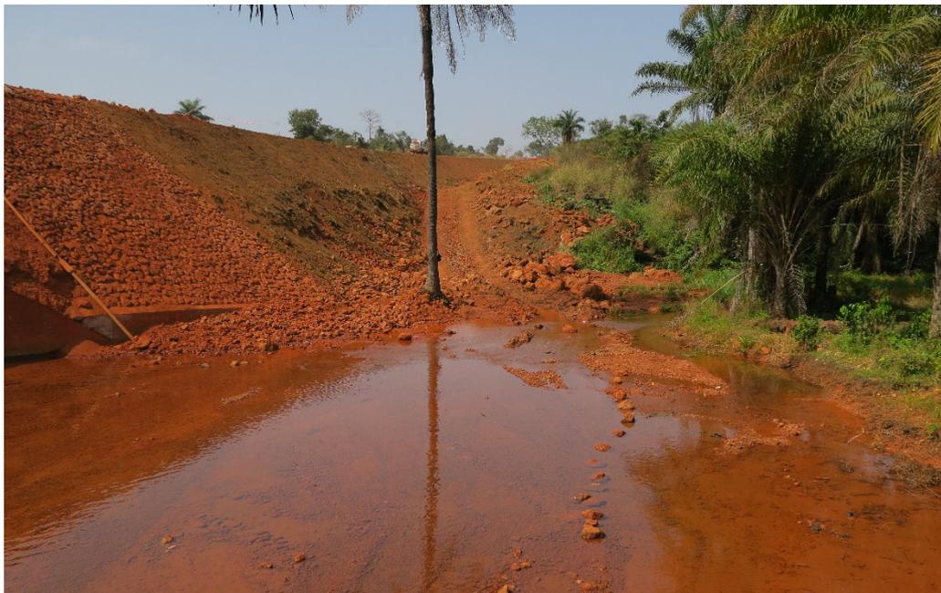
**Photo 34.** Thiapikour river crossing – poor erosion control/evidence of sedimentation
