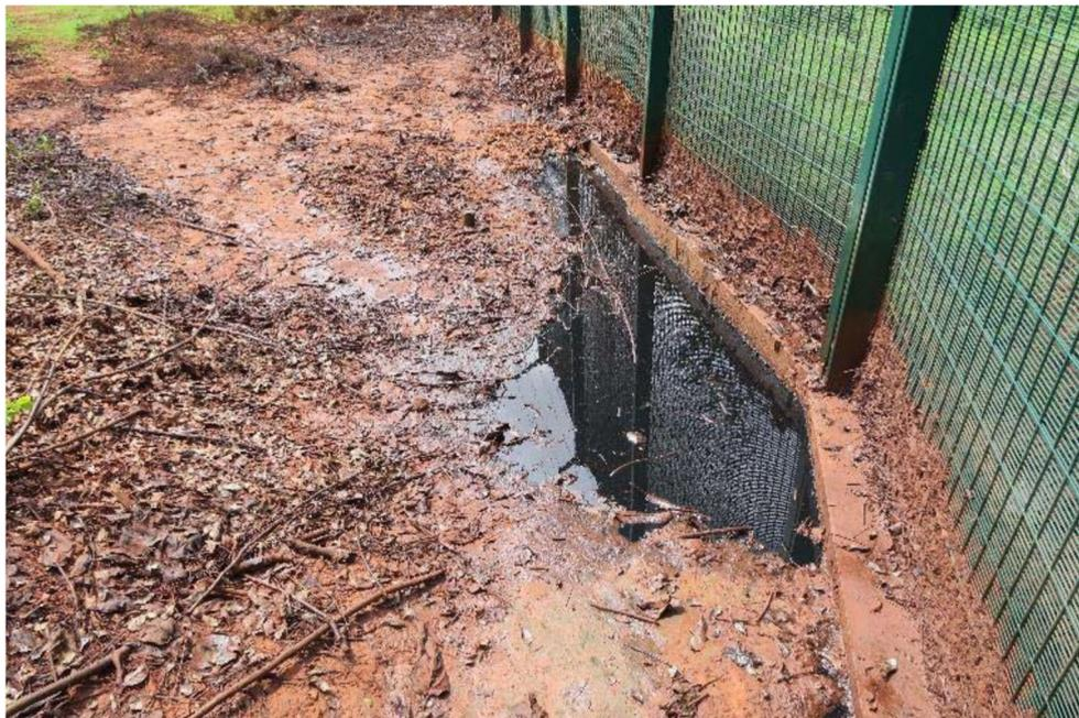
**Photo 29.** Feb 2018 – blocked drainage channel and accumulation of oil at Sangaredi workshop boundary fence
