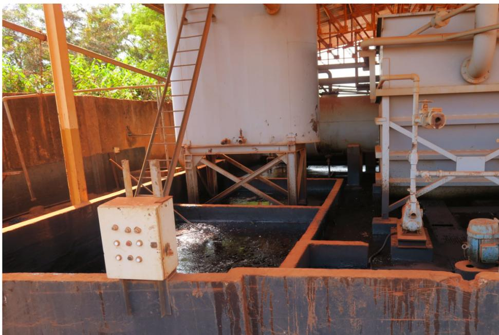
**Photo 18.** Heavy oil contamination at decommissioned oil water separator
