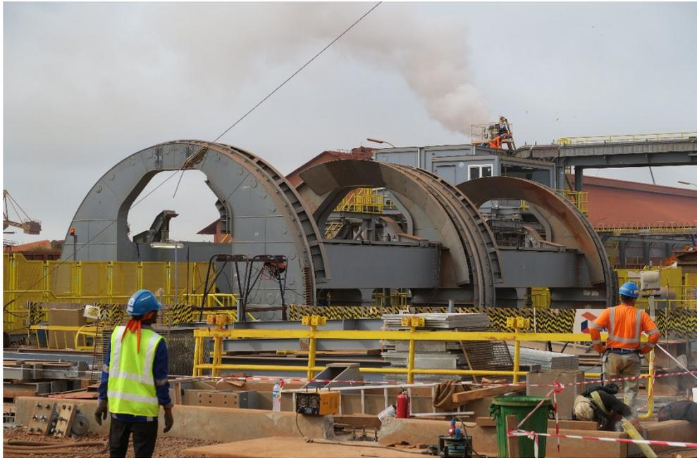
**Photo 1.** Newly constructed dual wagon tippler
