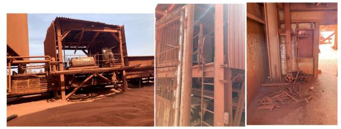
Figure 6-1 "Déferailleur" (Carter Missing or Defective) and Fire Hoses Broken on the Floor
