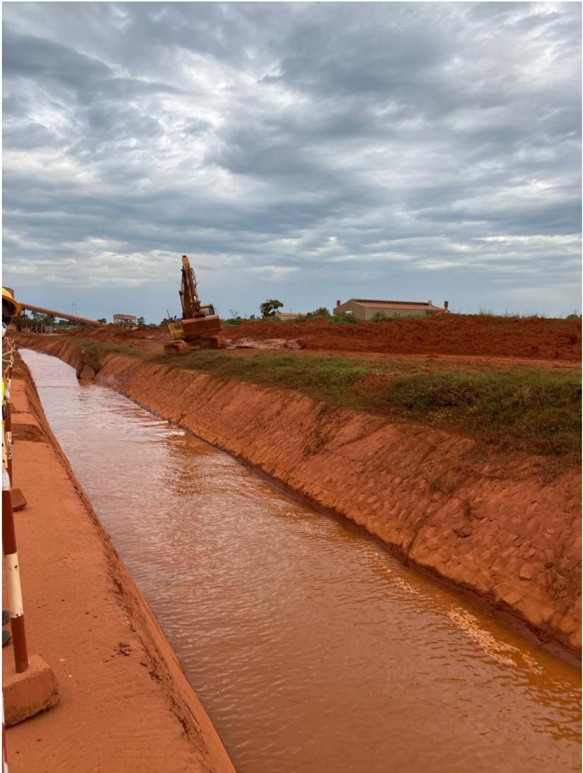
Figure 8-3: 'Grand Canal' (looking upstream) during cleaning (crane)
