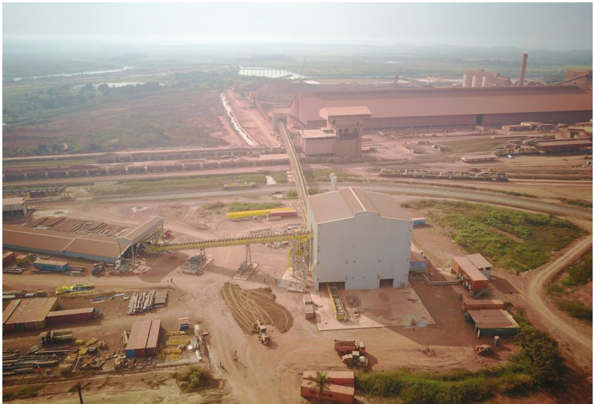
Figure 2: Operational conveyor belts and secondary sizer (courtesy of CBG)
