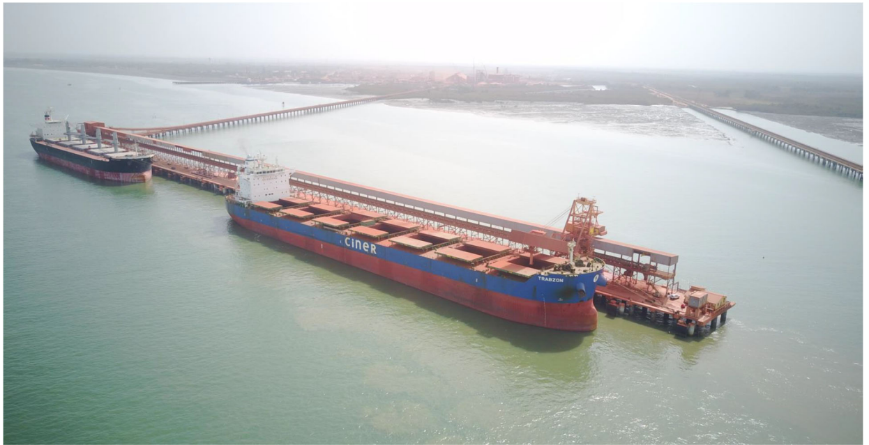
Figure 1: Extended jetty, capable of accommodating 2 bulk carriers (courtesy of CBG)
