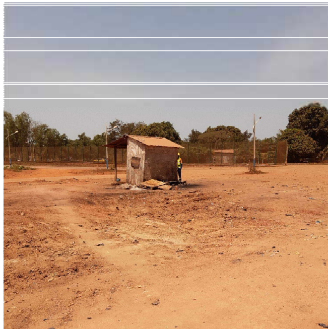
Photo 20. Security post at Tora Bora landfill
