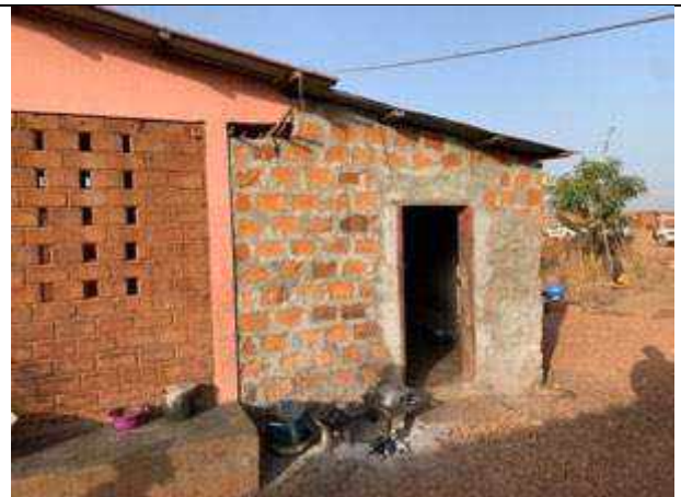
Addition of a kitchen to a resettlement house
