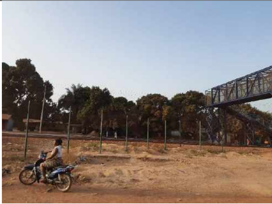
Photo 5. Fence posts awaiting completion with beta fence
