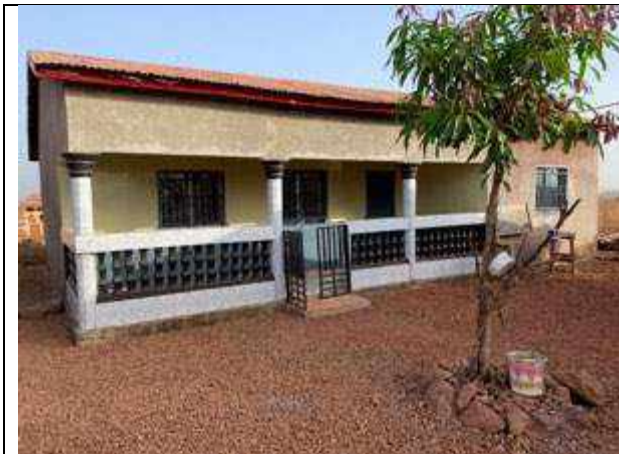
One of many new houses built by resettlers at the Hamdallaye resettlement site
