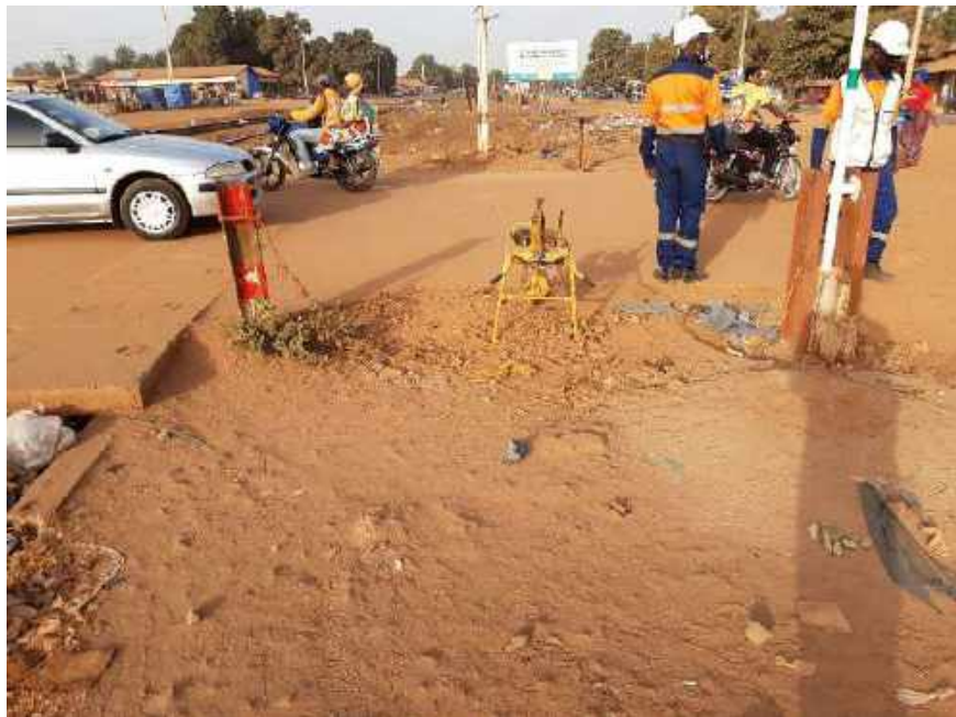
Photo 6. Level crossing manned by CBG. Note. Yellow klaxon to warn of approaching trains.
