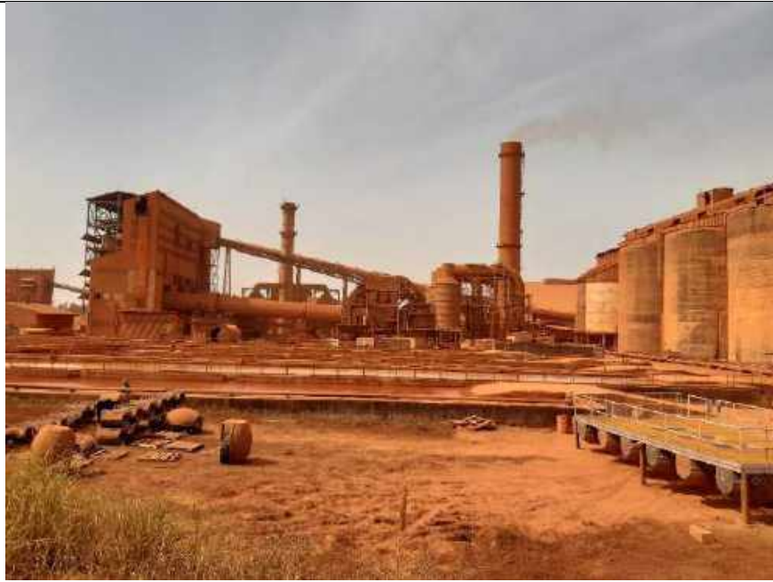
Photo 31. General view showing dryers and both dryer stacks (dryer 4 stack on the left)
