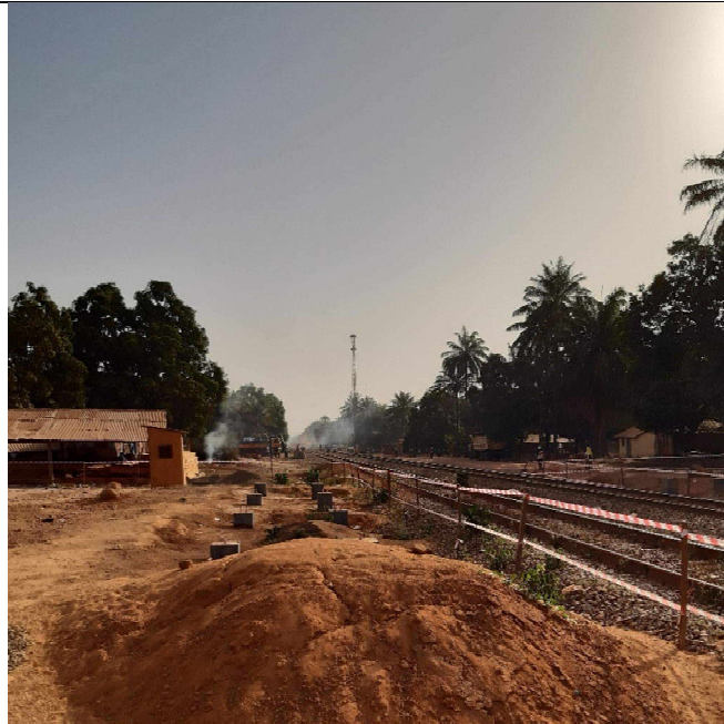
Photo 7. Earlier construction works for a footbridge at Kolaboui
