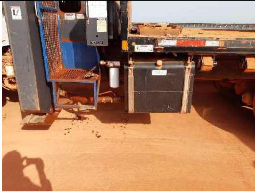
Photo 29. Poor maintenance of fuel hose on a vehicle resulting in loss of diesel on the jetty
