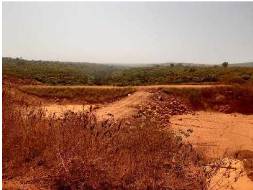
Photo 12. Retention basins intended to prevent sedimentation of a stream as a result of in mine site run off
