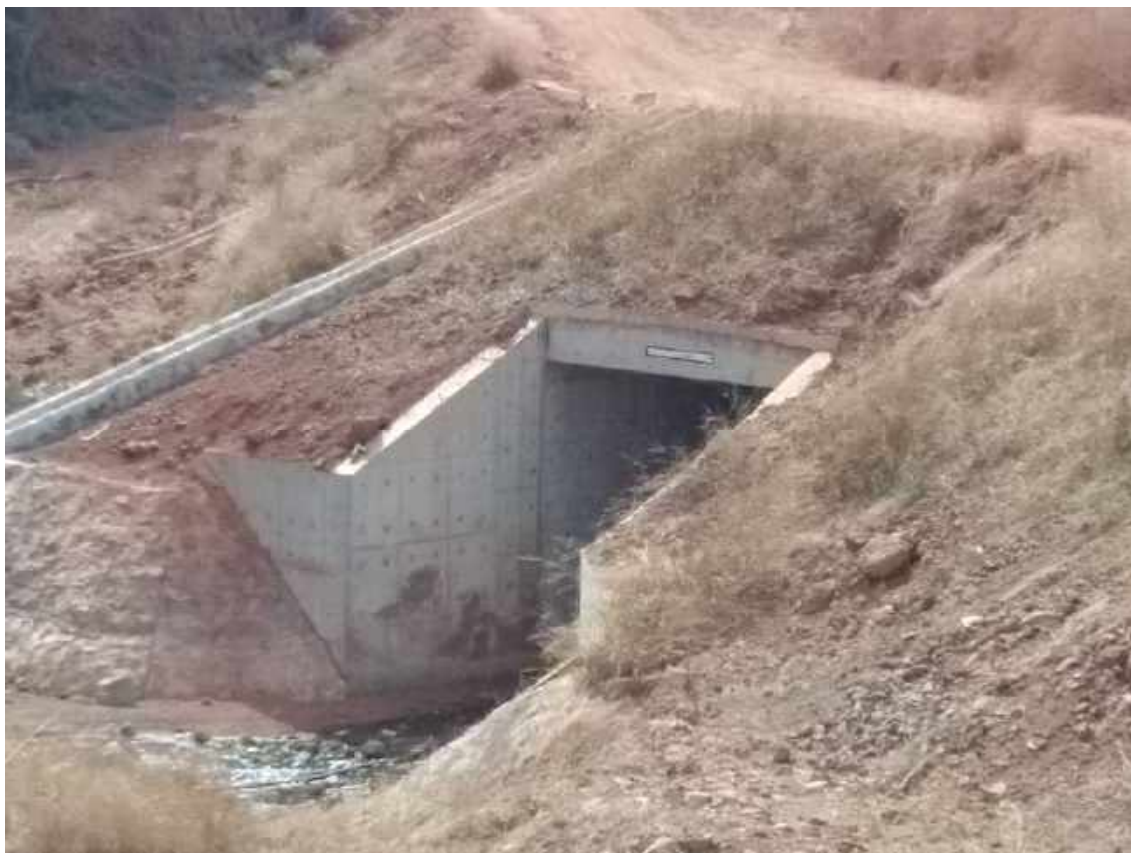
Figure 10-6: Small hydraulic crossing in the embankment of SMB-W railway
