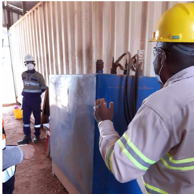
Photo 18. Fuel storage in location used as a refuge for operators at the waste facility.
