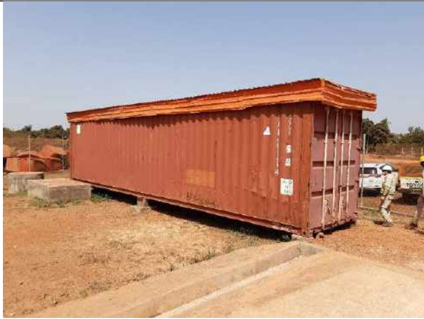
Photo 17. Office facilities at Tora Bora waste facility – awaiting commissioning
