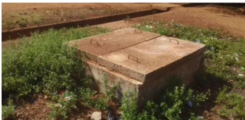
**Figure 7-9. Raised and repaired manhole cover to prevent rainwater ingress**
