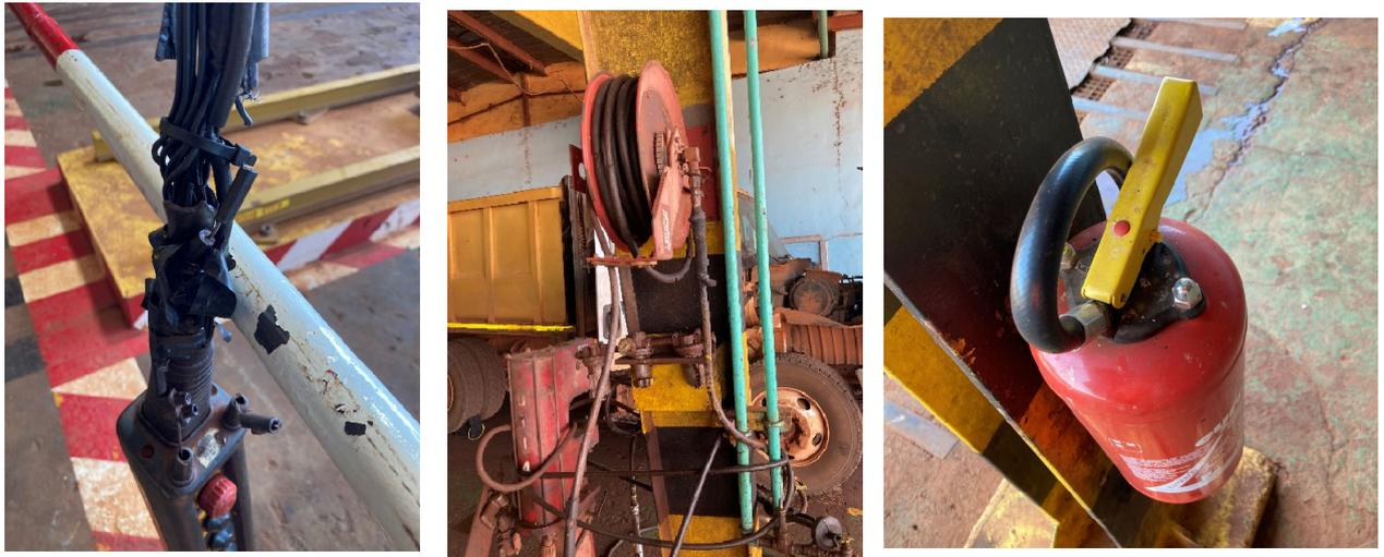
**Figure 6-4 Damaged controller module of a lifting device / fire hose cabinet out of order / extinguisher without safety pin**
