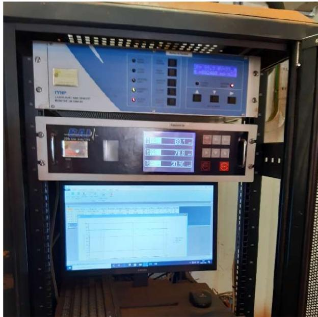
**Photo 11.** Control equipment for Continuous Emissions Monitoring equipment in dryer 4
