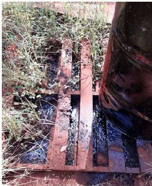
**Photo 8.** Loss of containment from oil containing free oil resulting in soil contamination
