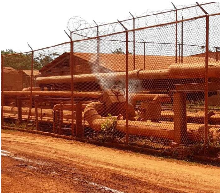
**Photo 12.** Steam from a leaking valve/damaged flange presenting risk to workers
