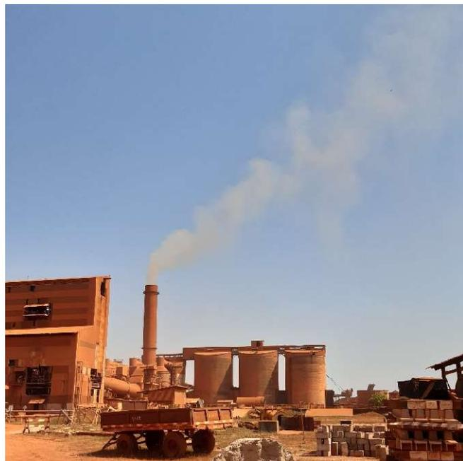
**Photo 6.** Visible dust plume from stack serving dryers 1 to 3
