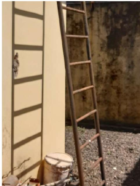
**Photo 13.** Inappropriate fixed ladder for access to roof at the air quality monitoring station, Kamsar
