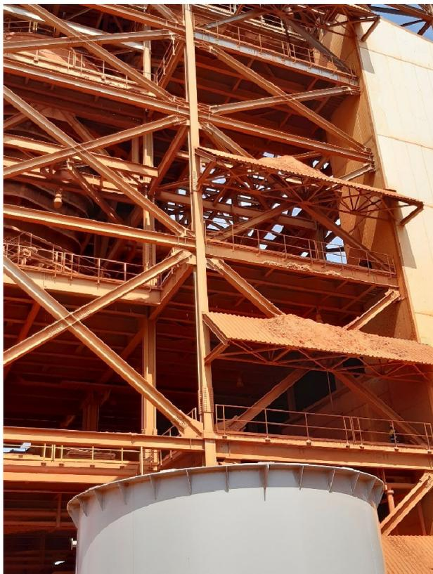
**Figure 6-3. Accumulations of dust above a working area**
