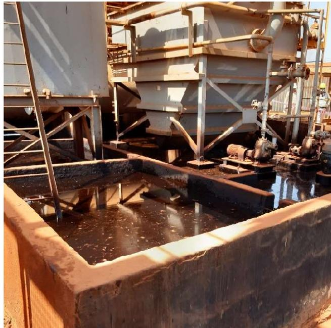
**Photo 9.** Risk of overtopping from old oil water separator due to ingress of rainwater
