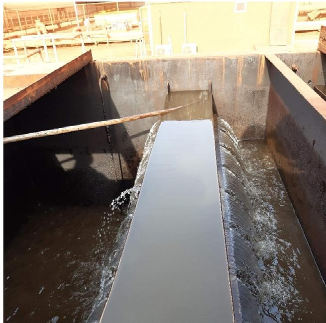
**Photo 30.** Oil water separator – treated water
