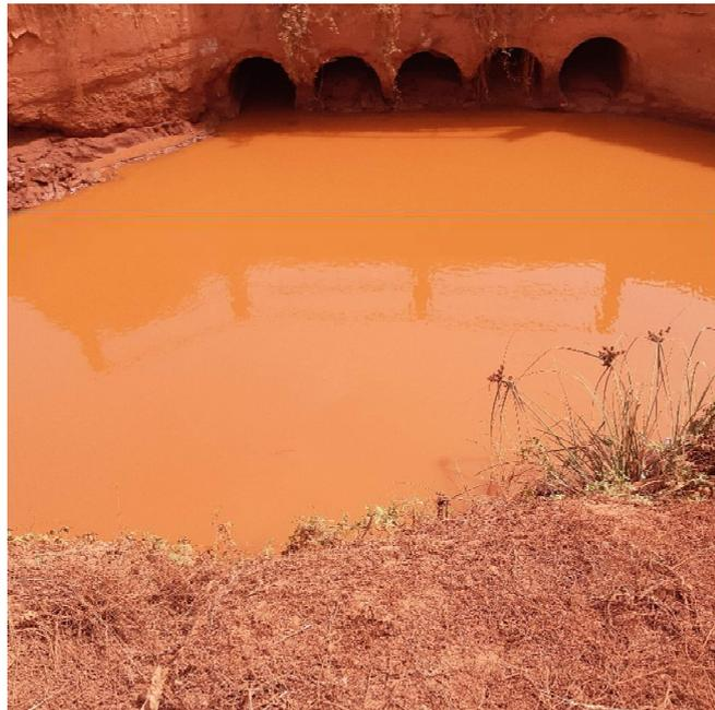
**Photo 24.** Heavily sediment laden discharge exiting CBG perimeter.
