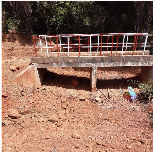
**Photo 10.** Poor construction practice adjacent to dried up stream. Earthworks resulting in soil being moved into the dry stream
